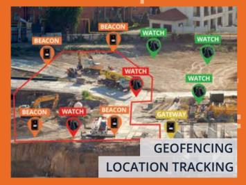
A single *R-Link* gateway located at the end of a beacon mesh or at the watch charging areas, automatically and safely transmits data to the powerful cloud-based Reactec Analytics software under GDPR compliance.
