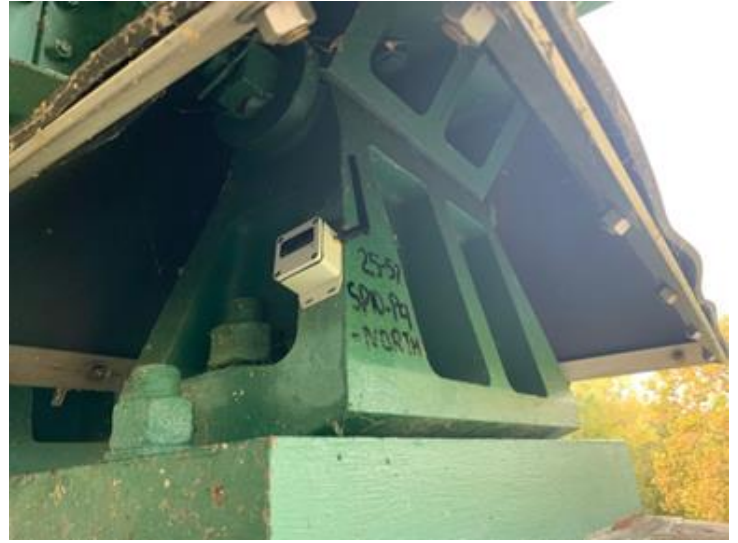
Resensys Wireless Tilt SenSpot™ sensor on bearing for monitoring bridge under superloads
