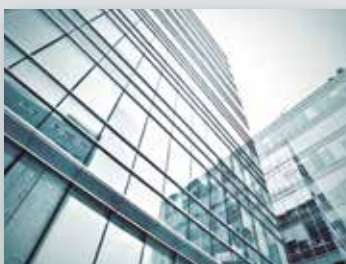
Measurements of acoustic insulation for airborne noise, impact noise and in façades
